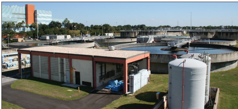
The Falkenburg Wastewater Treatment Plant in Brandon receives electricity directly from the County's Resource Recovery Facility next door, saving thousands of dollars each month.
